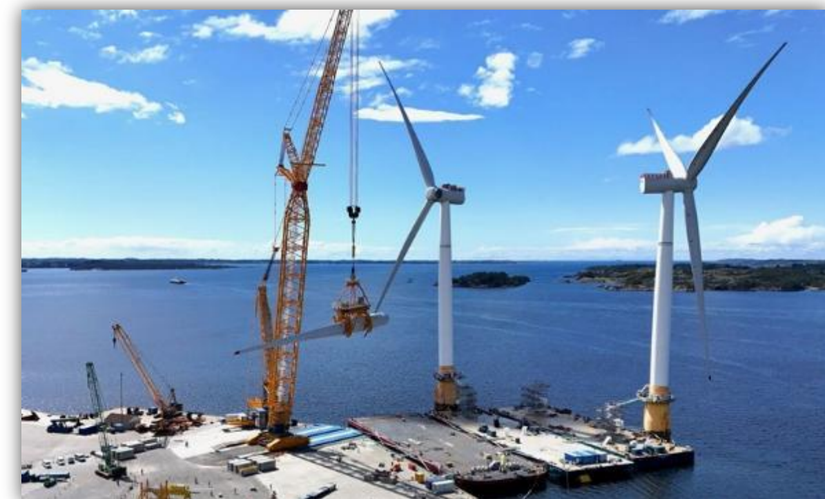
Offshore staging/ loadout [Hywind Scotland]
