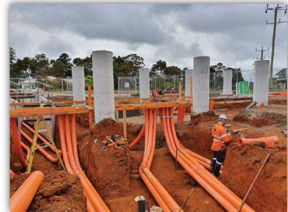
Substation civil works [Utility magazine]
